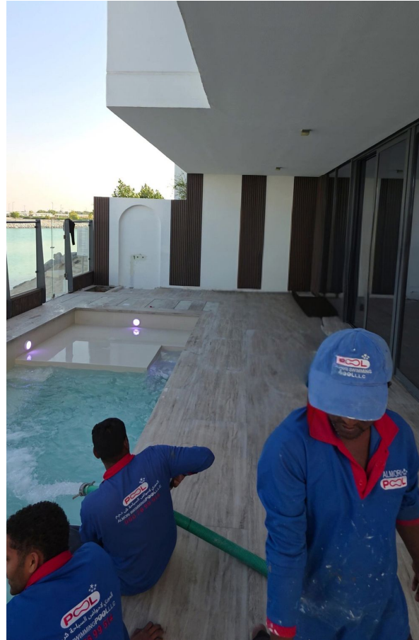
FINISHED POOL & GLAZED PANEL
