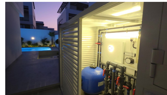
GARDEN POOL INSTALLATION
